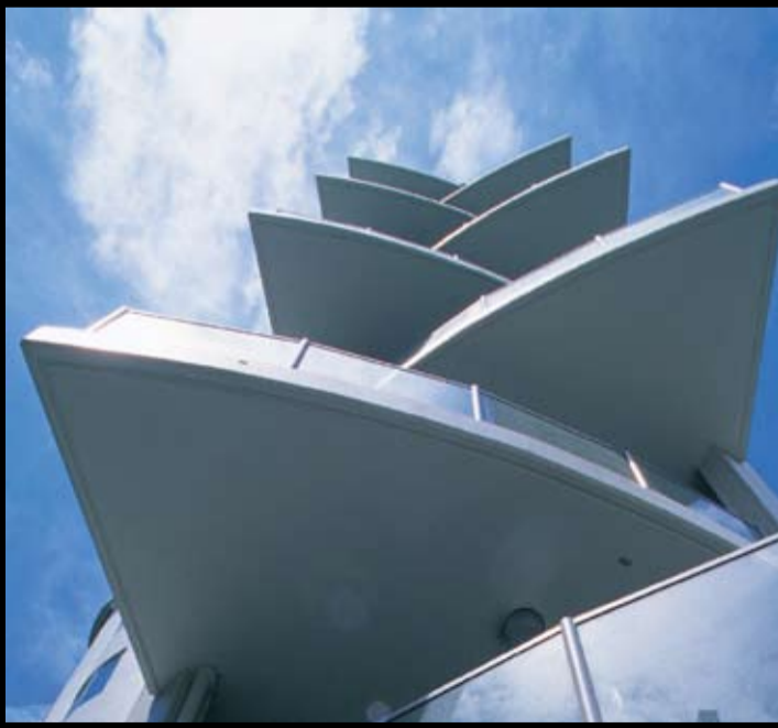
Figure 15. Waratah Mills-Adaptive Reuse
